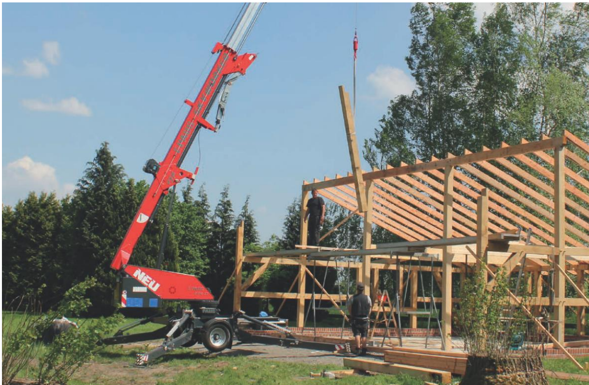
The Sky Worker PTK 27 aluminium trailer crane was developed especially for compact spaces
